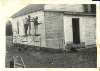
Figure 2: Neighborhood Youth Corps workers fixing up the Center.
